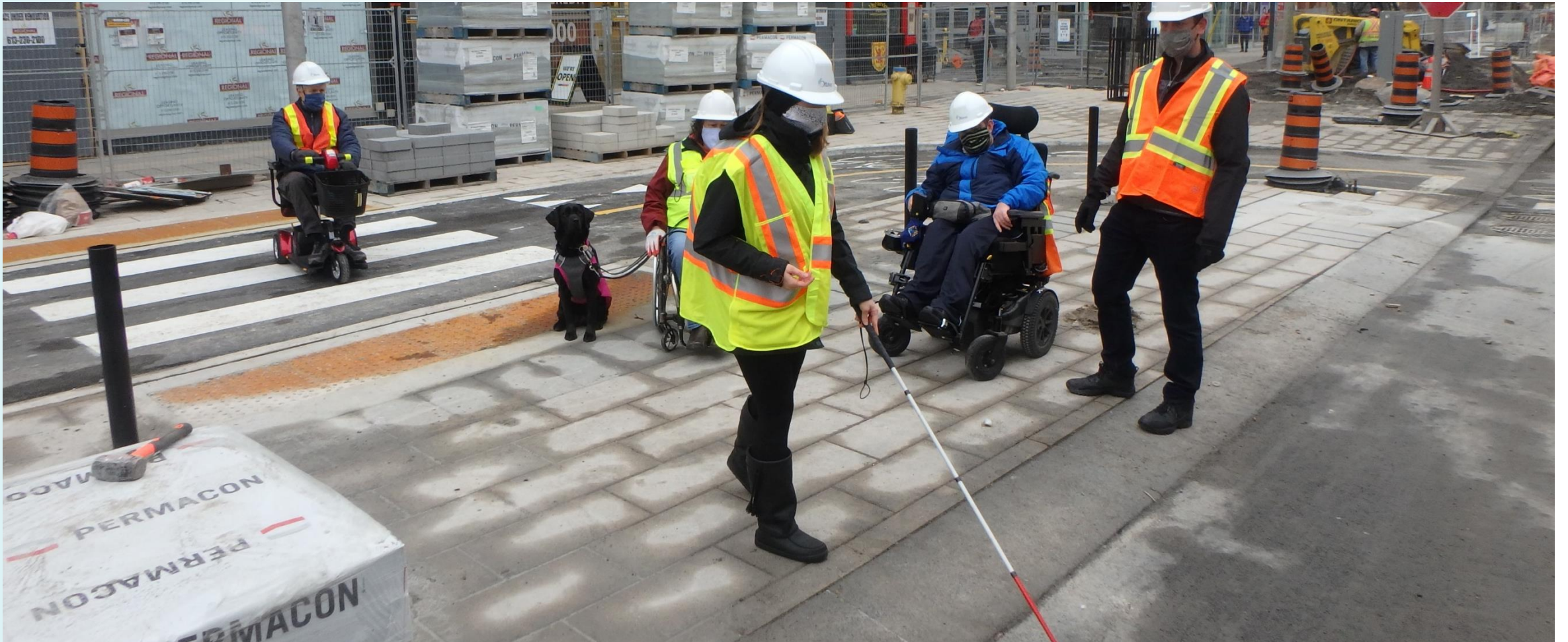
Angled curb testing on Rideau Street during Nov. 30 th on-site workshop
